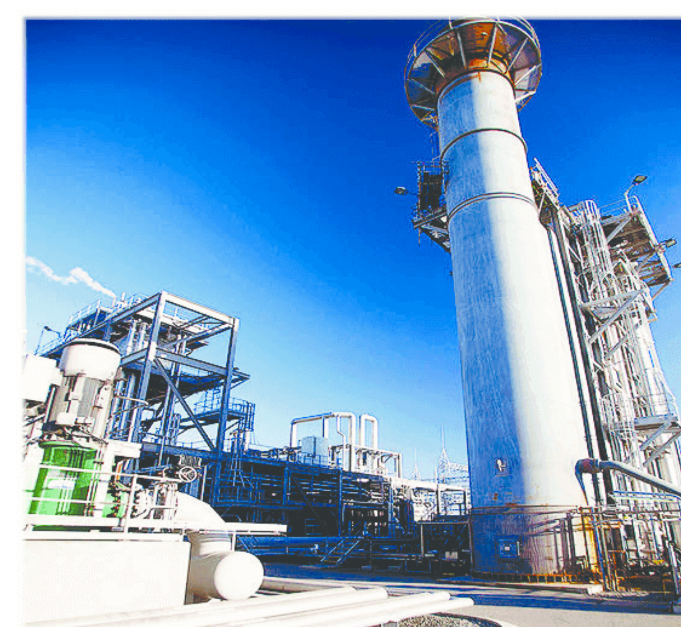
FIGURE 12 The Kwinana Cogeneration Plant is primarily fuelled by natural gas from Western Australia's gas fields, north of Perth. This cogeneration plant supplies otherwise waste steam directly to the nearby BP Australia Kwinana Oil Refinery. Also its proximity to the refinery minimises energy loss due to transmission distances. The remaining electrical energy is supplied to the state grid.
